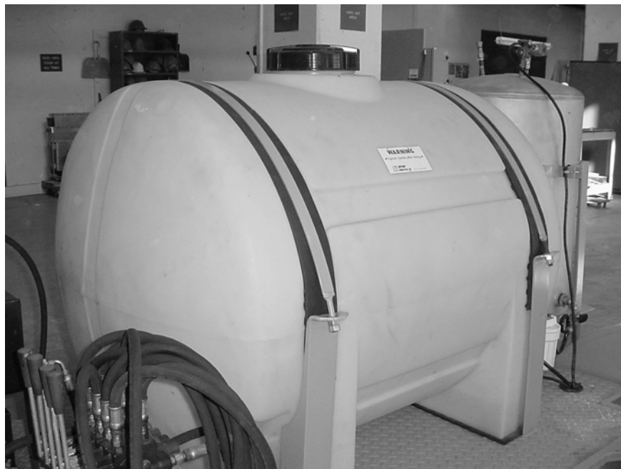
Figure 3-2: One of two water tanks.
