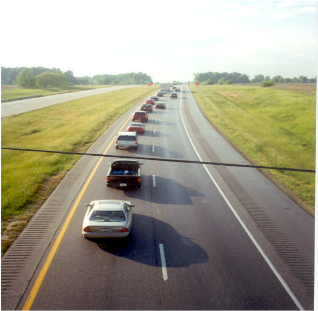
Figure 5.2: North bound side of the construction zone (MP 180 near US 43 interchange)
