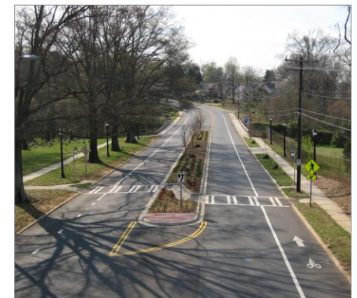
ABOVE: Distinct bicycles lanes, pedestrian crosswalks, and pedestrian havens enhance safety and are a key component of a strong, complete transit system.
