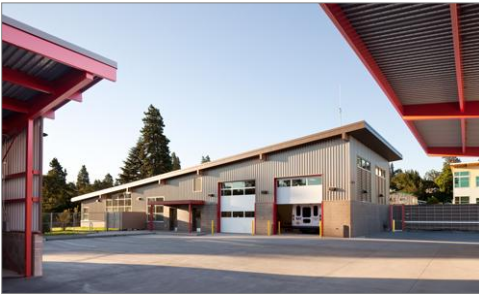
ABOVE: The Hood River Transit Maintenance facility funnels vehicles to the back of the site leaving the front of the facility as a public face for the district. Photo credit: Pivot Architecture
