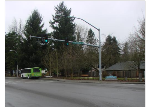
ABOVE: Example of far side bus turn-out. Lane Transit District suggests the "...use [of] the intersection itself as part of the far-side turn-out. This provides an easy pull-out for the bus, allowing the bus to get out of the highway traffic, and gives it protection when it pulls back into traffic, especially if the intersection is signalized." Photo credit: SMART
