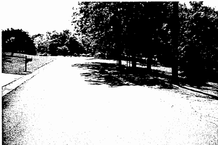
Figure 20. Oak Hill Drive – Underlying centerline joint reflected in FB-3.
