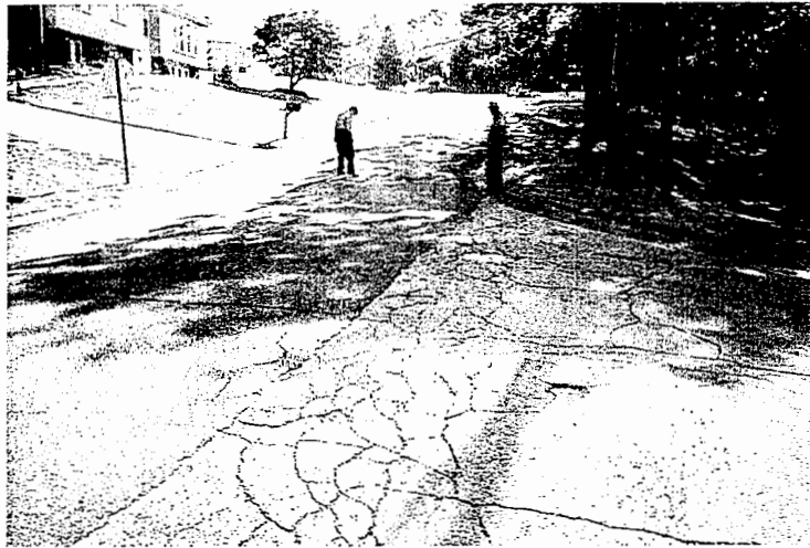
Figure 27. Oak Hill Drive - Reflection cracking in FB-3 Modified surface (on left) at the intersection with North View Court (on right).
