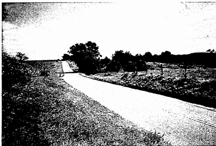
Figure 23. Rinely Road test section 1 - Overall appearance from far end looking towards origin.
