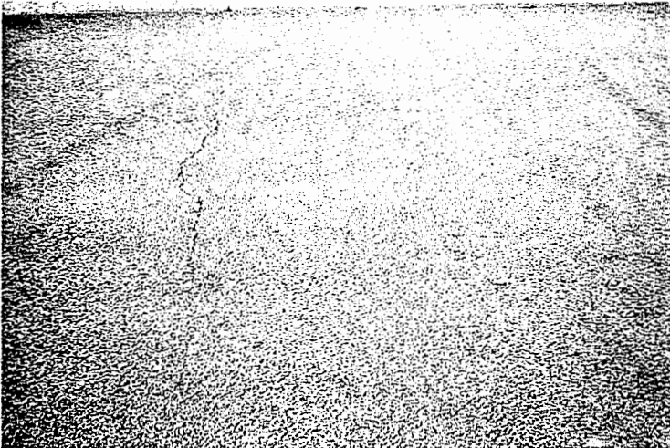
Figure 26. Oak Hill Drive - Transverse crack in center of roadway where ends of crack have healed.
