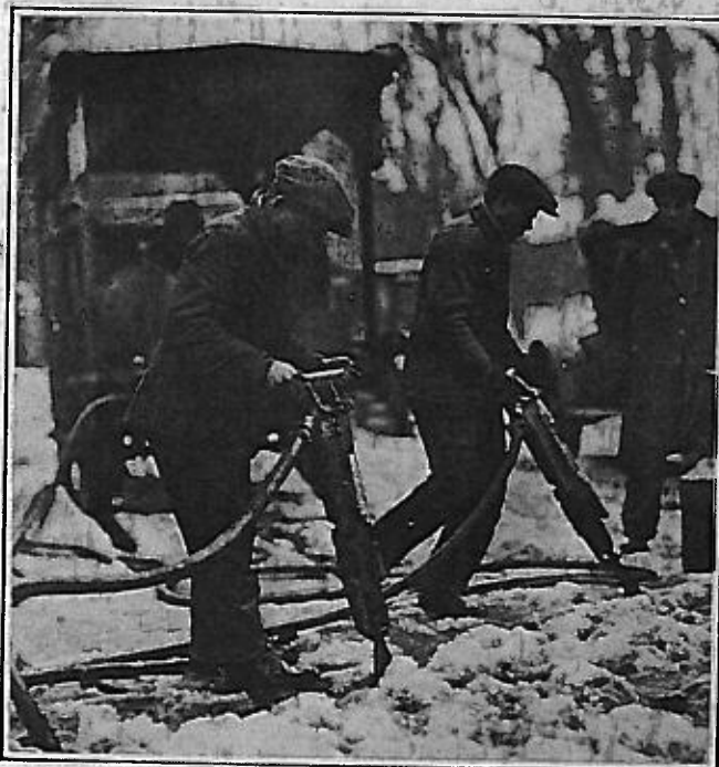
Pneumatic Pavement Cutters Break Up Ice in Buffalo, N. Y.
