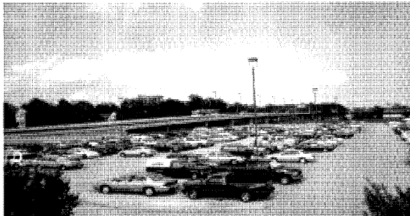
Freeway Park-and-Ride Lot in Houston, Texas with a direct transit ramp connection.
