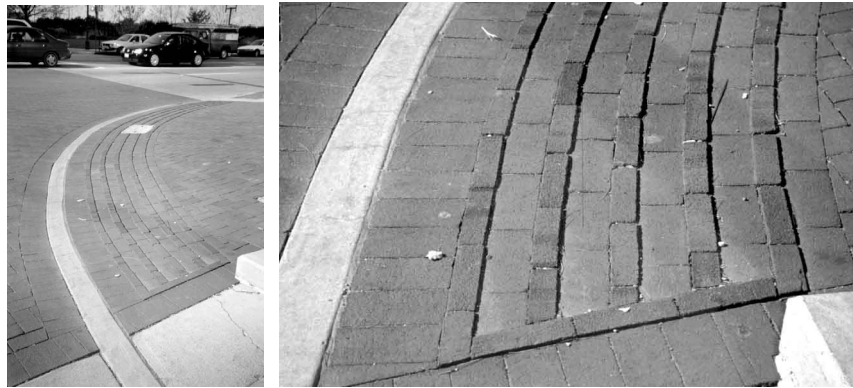
FIG. 1-3. A BLENDED CURB IN COLUMBUS, OH, WHICH USES DIFFICULT-TO-DETECT ROWS OF RAISED BRICK.
