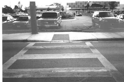
FIG. 5-6. MID-BLOCK CROSSING WITH CURB RAMP, AUSTIN.
