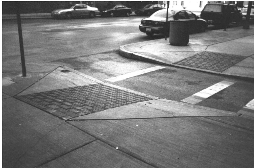
FIG. 1-8. CURB-RAMPS WITH TRUNCATED DOME DETECTABLE WARNINGS ON OPPOSITE SIDES OF AN ALLEY, CLEVELAND, OH.
