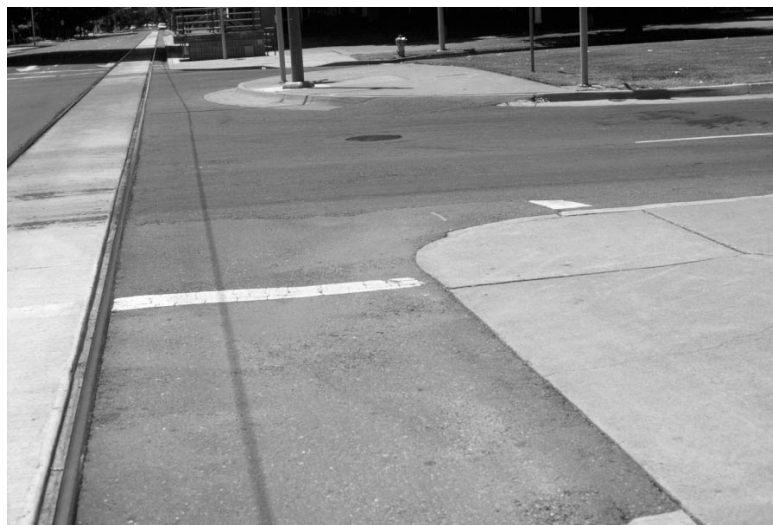
FIG. 3-1. WHERE THERE IS NO DIFFERENCE IN SLOPE OR ELEVATION BETWEEN THE SIDEWALK AND STREET, IT IS PARTICULARLY DIFFICULT FOR PEDESTRIANS WHO ARE BLIND TO DETERMINE WHEN THEY HAVE REACHED AN INTERSECTING STREET. BLENDED CURB IN SACRAMENTO, CA.
