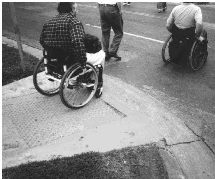
FIG. 3-2. STAMPED CONCRETE DETECTABLE WARNING ON CURB RAMP, AUSTIN, TX.
