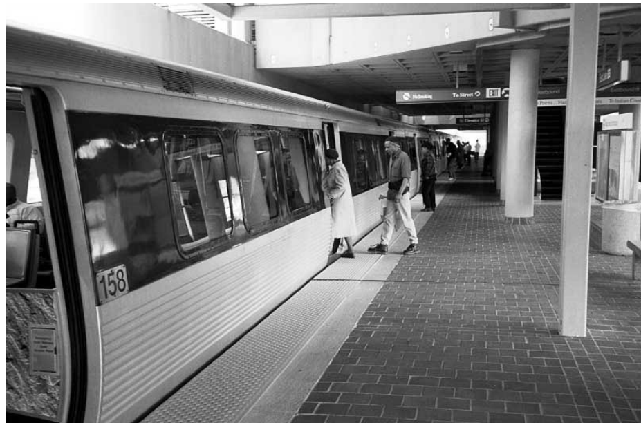
FIG. 5-8. MARTA STATION SHOWING INSTALLATION OF ARMOR-TILE.
