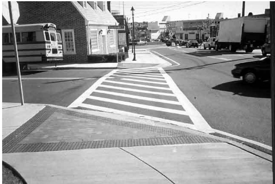
FIG. 5-14. A BAND OF DETECTABLE WARNING PAVERS OUTLINES THE TRIANGULAR SHAPE OF THIS CURB RAMP IN TOWSON, MD.
