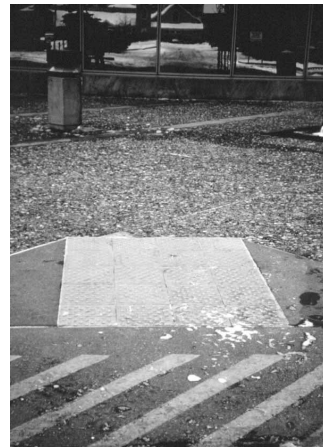
FIG. 5-3. (LEFT) CURB RAMP IN ANCHORAGE, AK.
