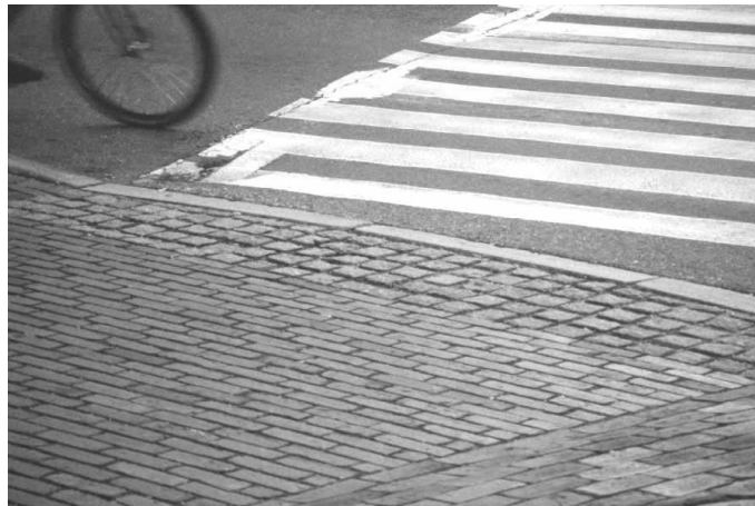
FIG. 5-1. A MINIMALLY DETECT- ABLE WARNING SURFACE IN PORTLAND, ME.
