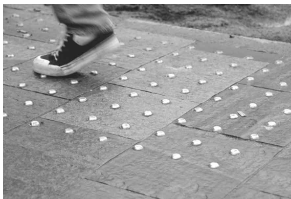
FIG. 4-4. BRASS NAILS INSTALLED IN PAVEMENT AS DETECTABLE WARNINGS.
