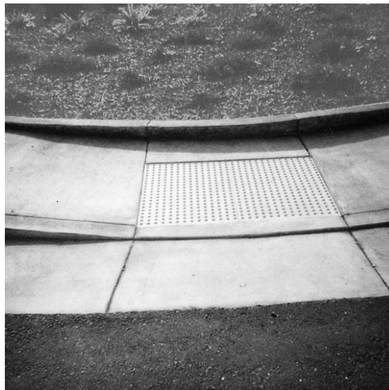
FIG. 5-10. PARALLEL CURB RAMP IN ROSEVILLE USING ARMOR-TILE PANEL.
