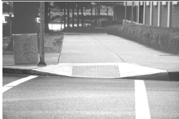
FIG. 5-11. BRICK DETECTABLE WARNING SURFACE CONTRASTS WITH ADJACENT CONCRETE, HARRISBURG, PA.
