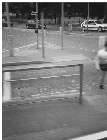
FIG. 3-6. (LEFT) DETECTABLE WARNINGS (BLISTER SURFACE) ON THE THREE CURB-RAMPS AT A SPLITTER ISLAND, IRELAND
