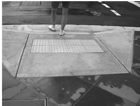
FIG. 4-5. (LEFT) AUSTRALIAN CURB RAMP WITH DETECTABLE WARNING.
