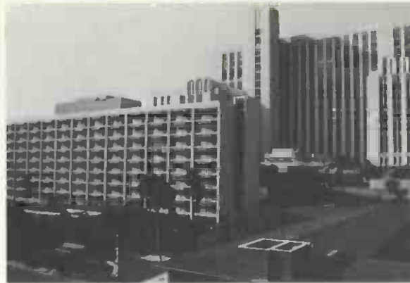
LA County Hospital
