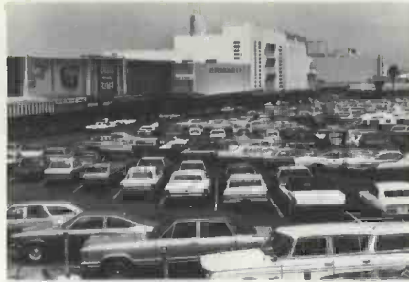
Crenshaw Shopping Center
