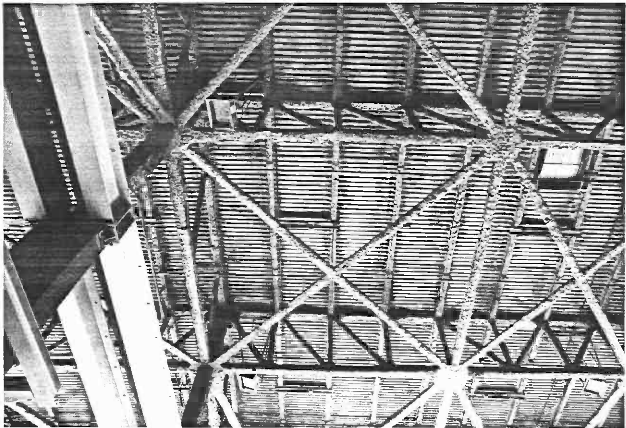
RM. 124- ROOF TRUSSES, BOT. CHORD BRACING & PURLINS.
