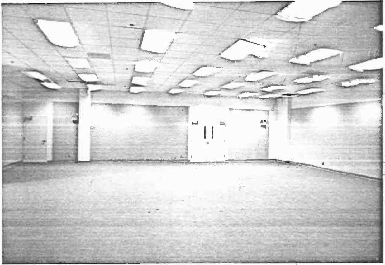
RM. 245- GWB WALL FINISH W/ SUSPENDED ACOUSTICAL CEILING.
