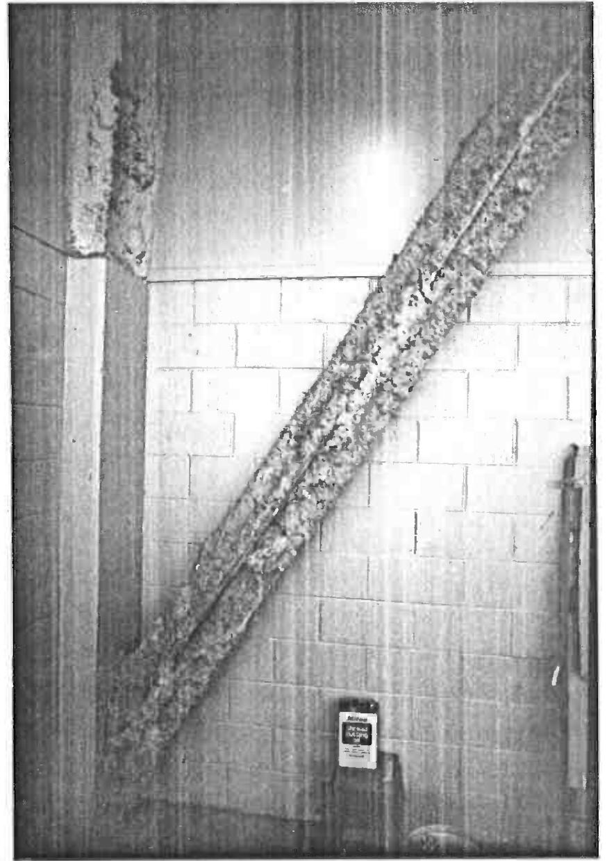
RM. 104- COLUMN F.6-6 W/ K-BRACING
