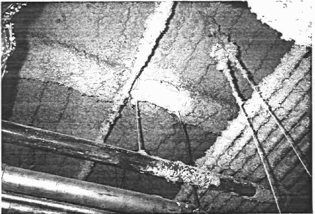
RM. 249- ROOF DECK FIREPROOFING PATCHED WITH MONOKOTE.
