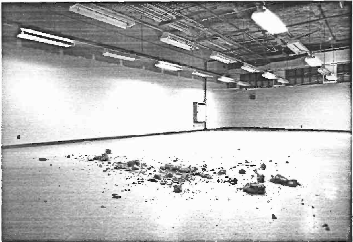
RM. 249- FIREPROOFING ON FLOOR.
