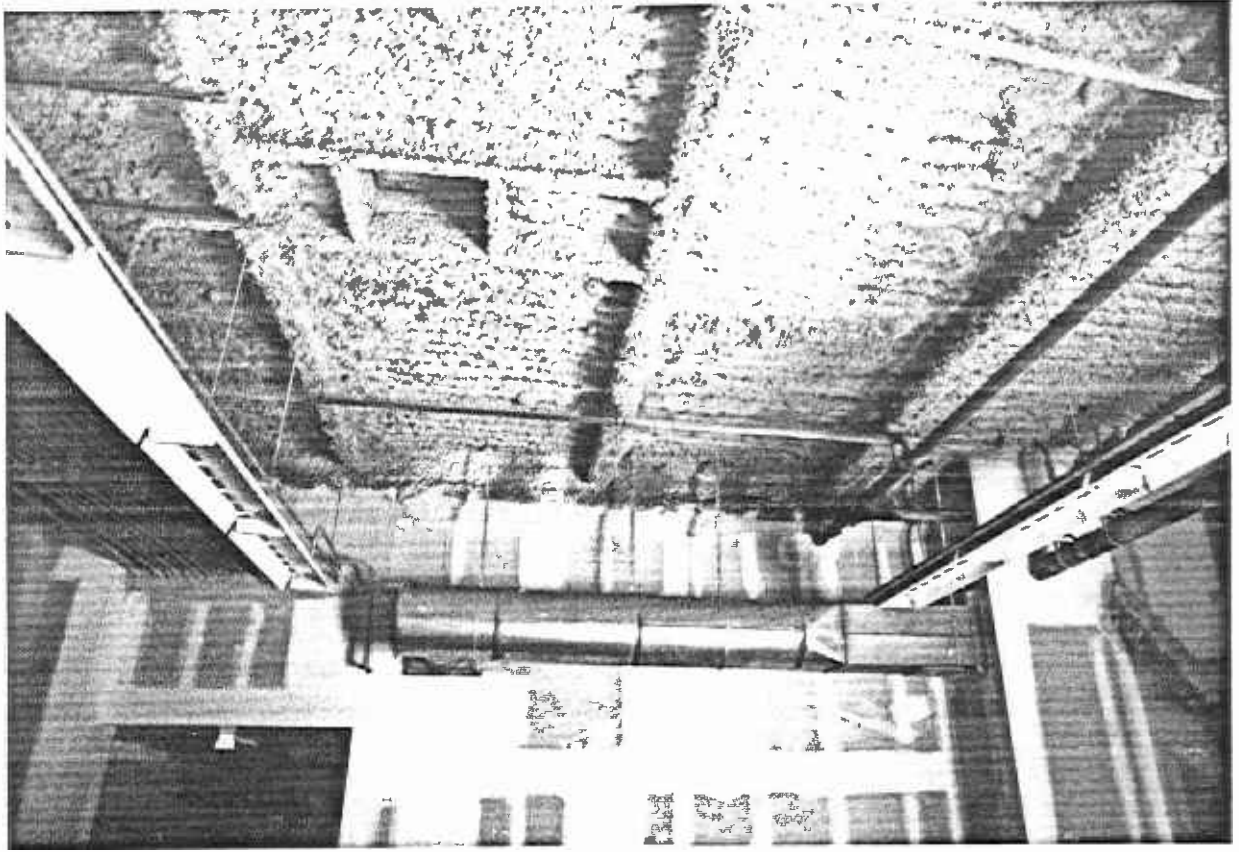
RM. 278- EXPOSED ROOF DECK
