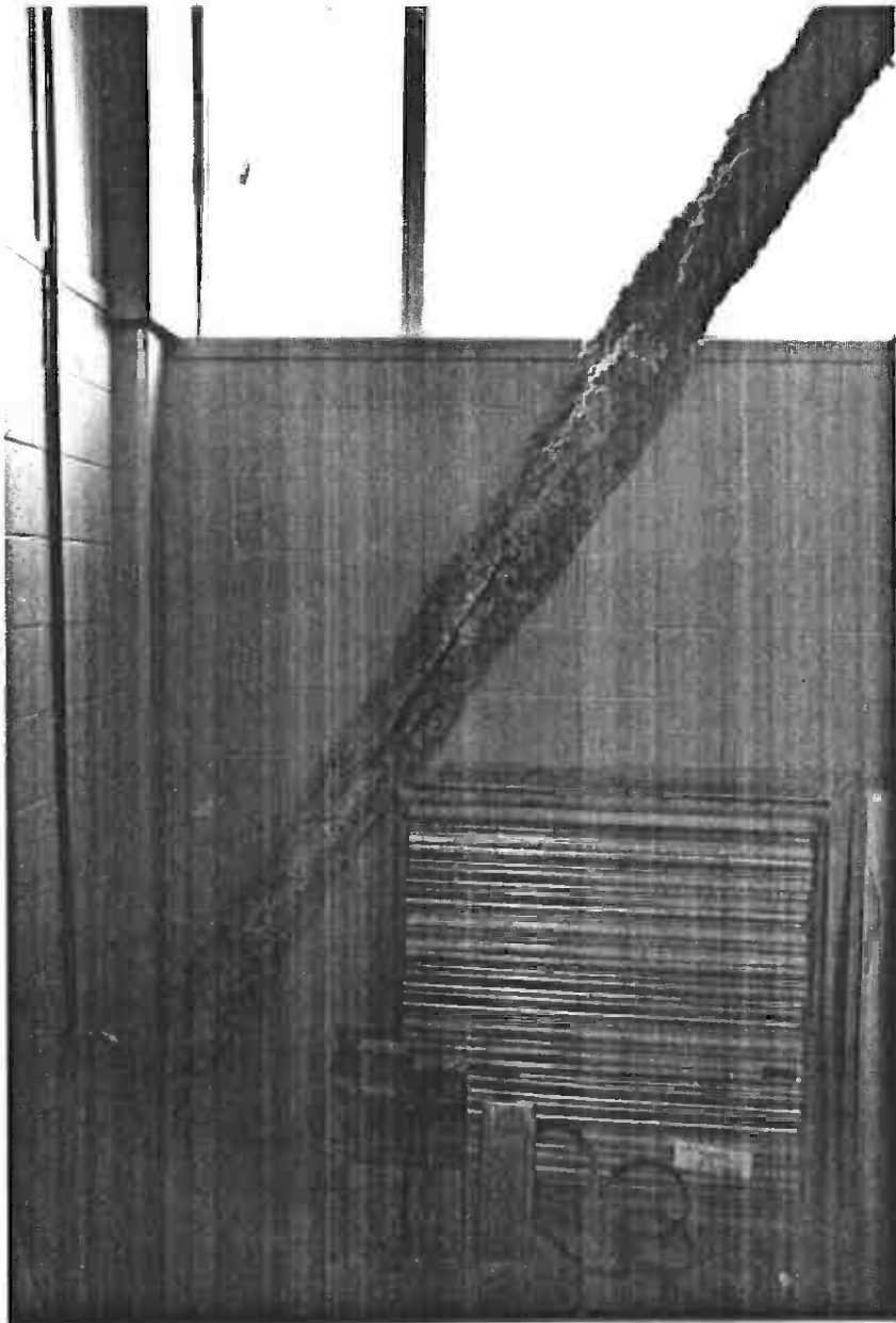
RM. 104- COLUMN G-7 W/ K-BRACING
