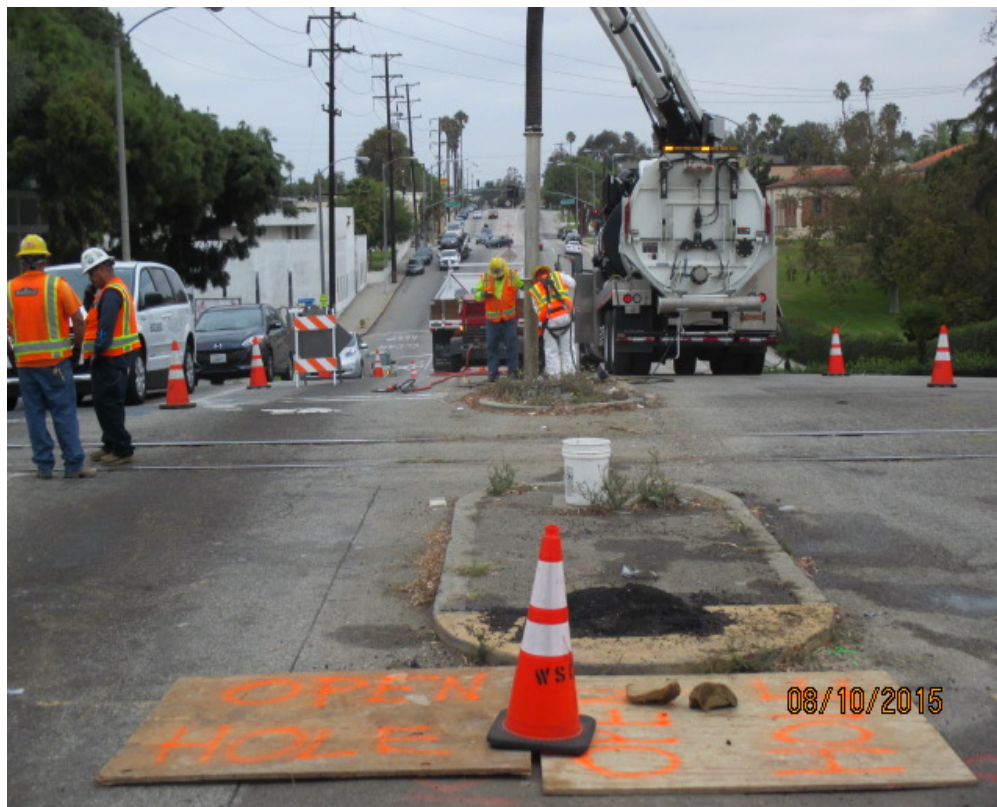
CENTINELA – Utility potholing on the north end.
