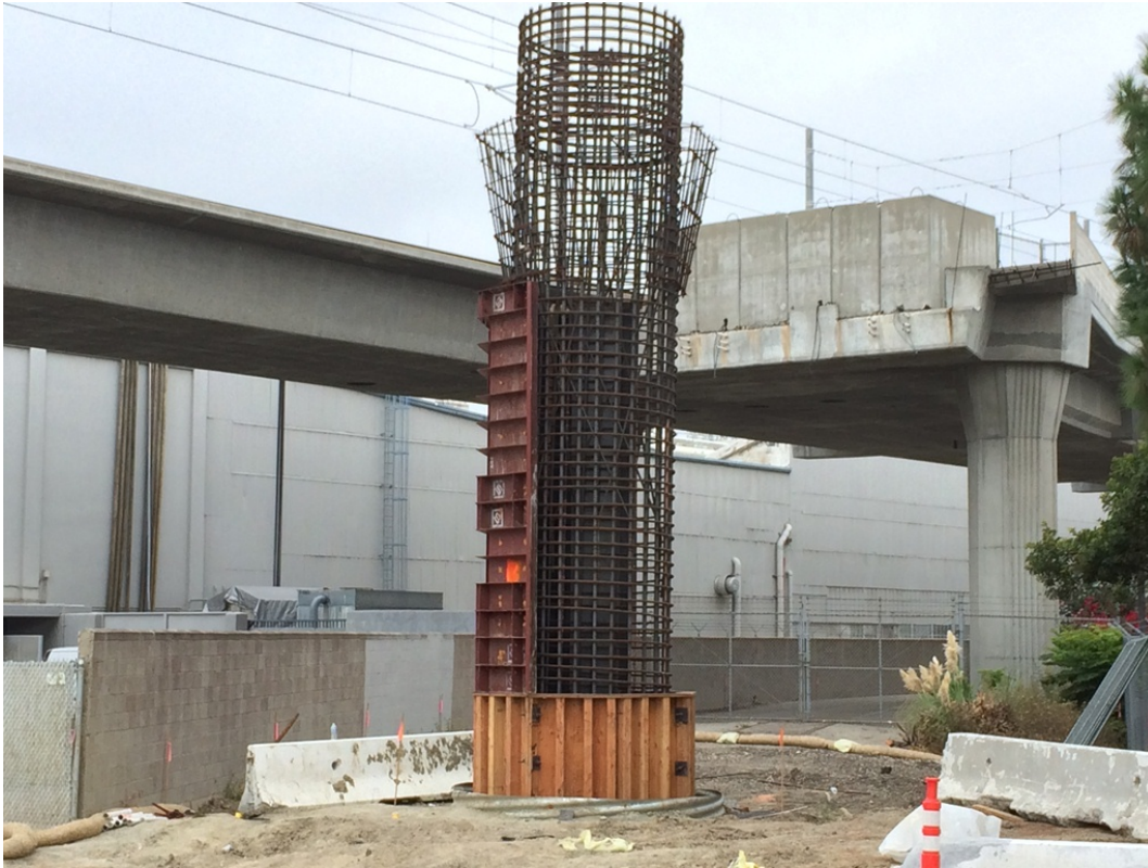
GREEN LINE - Underpass Bent 1A Column Formwork Placement.
