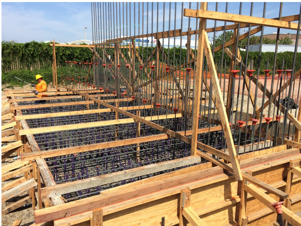
GREEN LINE – Underpass Abutment 6 Footing.
