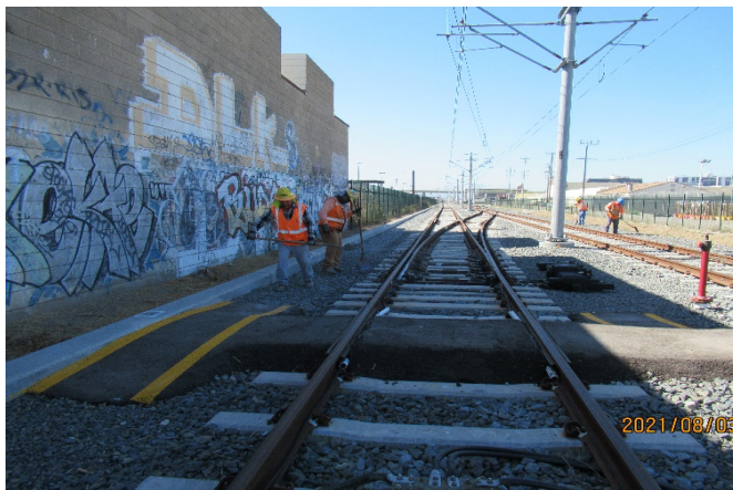
AVIATION STATION – NB track near STA 103+10 Segment A, adding & dressing walkway ballast on right side shoulder
