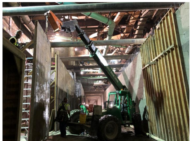
Form installation for west interior track wall at Flower St
