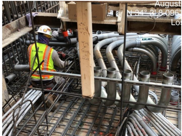
Conduit installation at Ancillary Level at Historic Broadway Station
