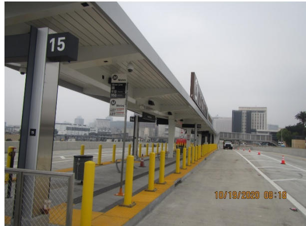
Finishing Canopy, placing sigs, cameras, and striping
