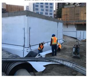
HDPE installation at the Equipment Access Shaft at Grand Av Arts/Bunker Hill Station
