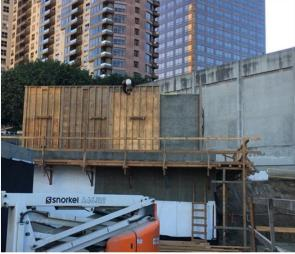
Stripping forms at the Upper Roof Level Tunnel Vent Shaft West at Grand Av Arts/Bunker Hill Station
