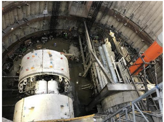
TBM Assembly in Tail Track Exit Shaft
