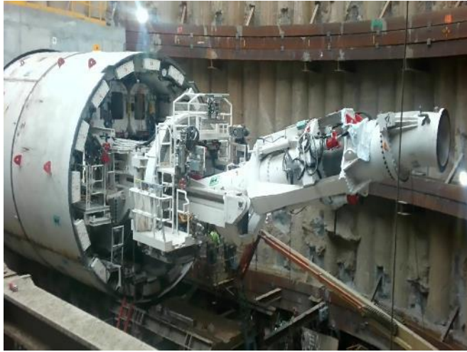
BL TBM Assembly at Tail Track Exit Shaft
