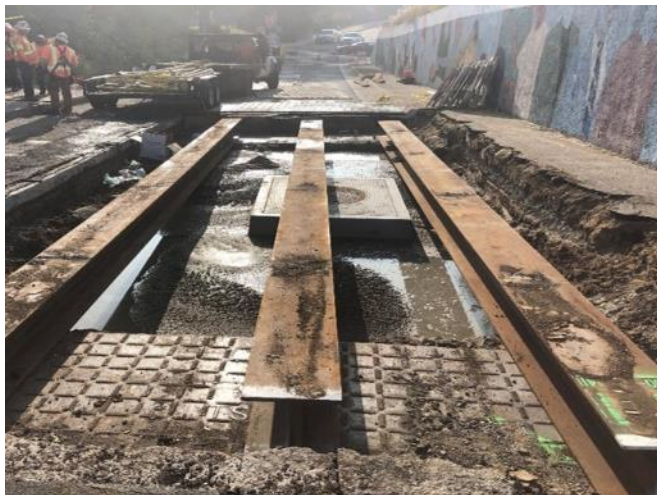
Installation of Underground Conduits to SCE Vaults near VA Campus
