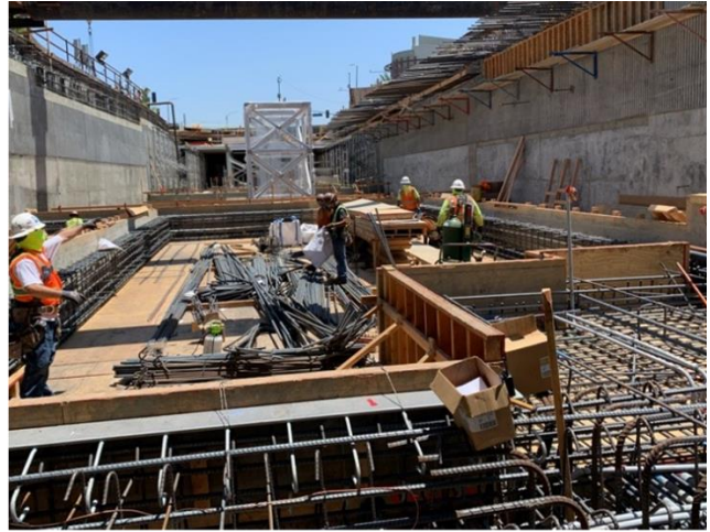
Installing forms at mid-landing of future Little Tokyo/Arts District Station
