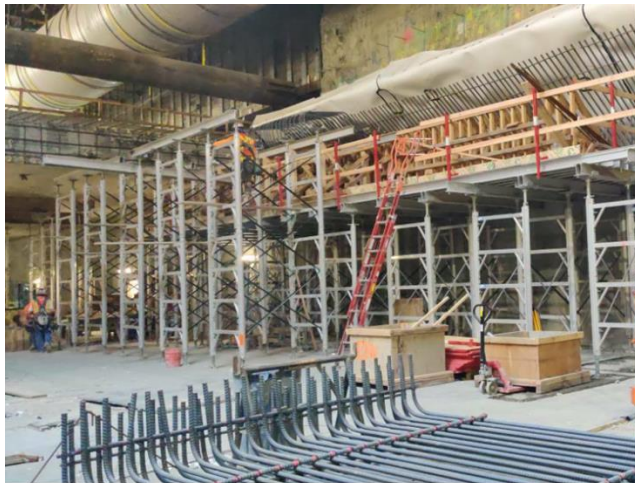
Roof deck shoring at Historic Broadway Station
