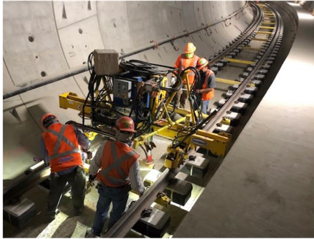
Setting rail height and aligning rail in Reach 3 RT
