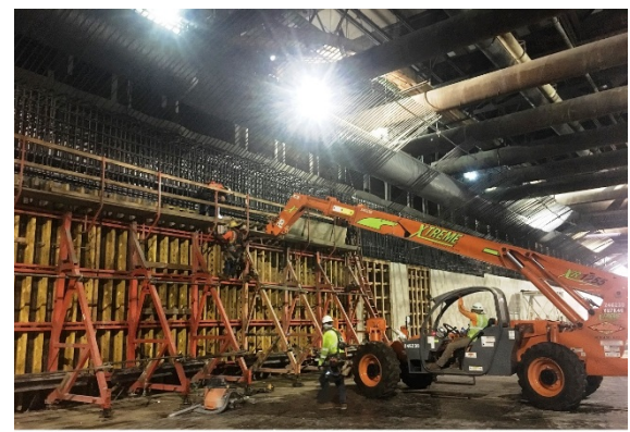
2 nd Lift Wall Formwork at Wilshire/La Cienega Station
