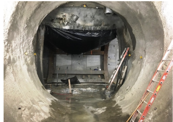
Reach 1 Cross Passage #8
