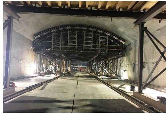
Wilshire/La Brea Station Arched Roof
