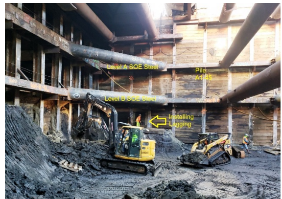
Entrance Apperage Excavation at Wilshire/Fairfax Station
