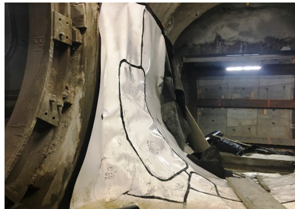
HDPE Application at Reach 1 Cross Passage #11
