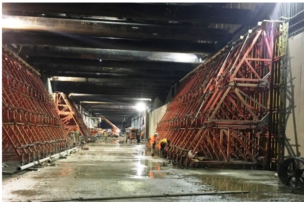
Exterior Wall Forms at Wilshire/La Cienega Station
