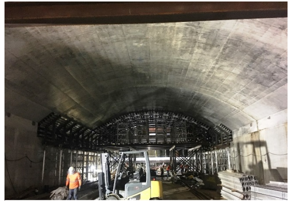
View of Roof Concrete at Wilshire/La Brea Station
