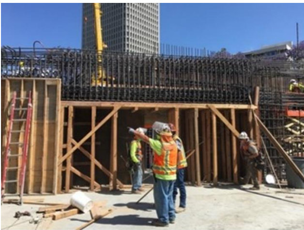
Forming roof level wall at Grand Av Arts/Bunker Hill Station
