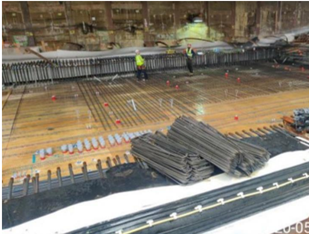
Bottom mat rebar installation at roof deck at Historic Broadway Station
