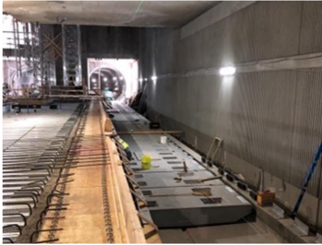
Floating slab at Grand Av Arts/Bunker Hill Station
