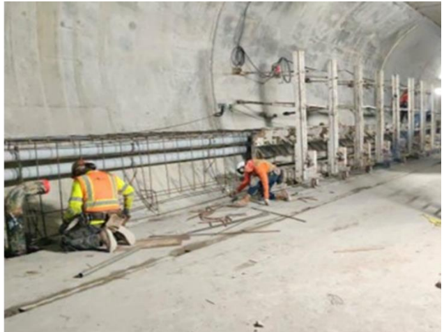
Emergency walkway installation in Crossover Cavern
