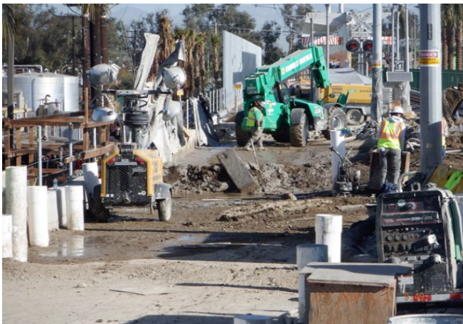
LA Brea Station – MSE Wall 202L repairs, jet grouting.
