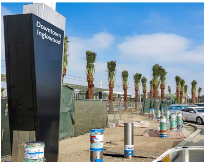
Downtown Inglewood- Station name pylon and safety steel bollards Installed.
