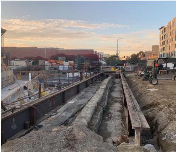
Removal of diagonal support and diaphragms at Central Ave
