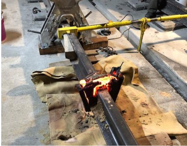
Rail welding in Reach 3 right tunnel
