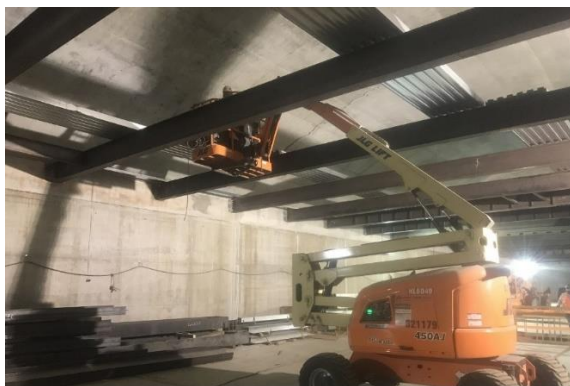
Installation of Plenum Beams at Wilshire/La Brea Station
