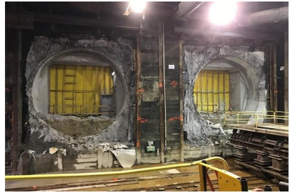
Knockout Panels Removed at Wilshire/Western Station
