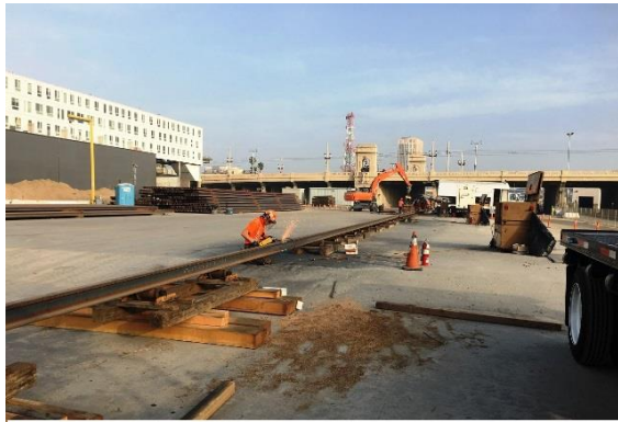
Checking Welded Rail at Division 20 Rail Yard
