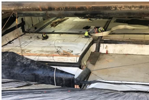
HDPE Placement at Wilshire/La Cienega Station
