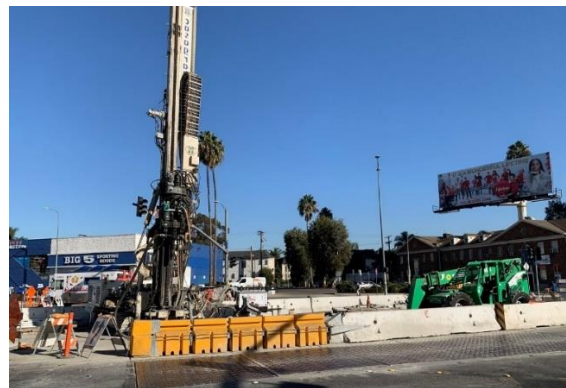
Reach 3 Anomaly Work at Wilshire/San Vicente
