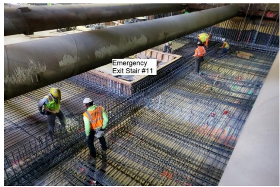
Concourse Rebar Installation at Wilshire/Fairfax Station
