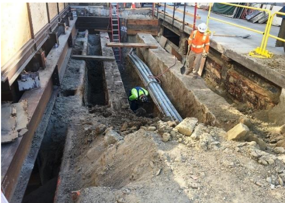
Excavation at Wilshire/La Brea Station Appendage
