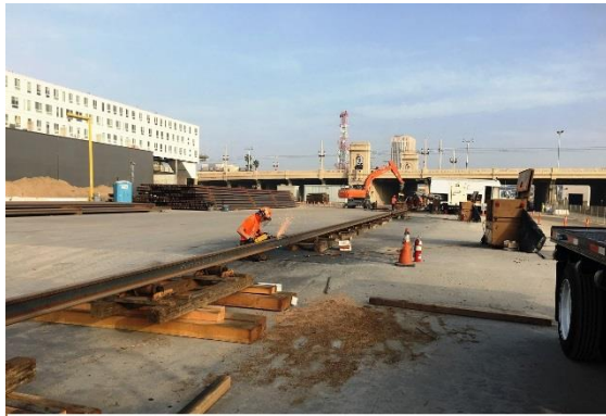
Grinding Welded Rail at Division 20 Rail Yard
