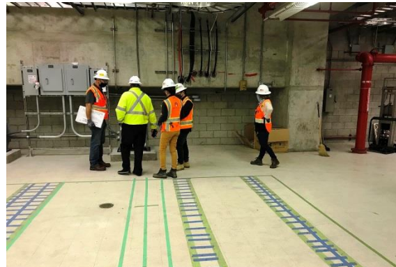
Surveying Electrical Equipment at Wilshire/Western Station
