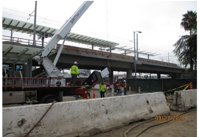
104 th Street – Erecting Grand Pylon sign at the Aviation Station
