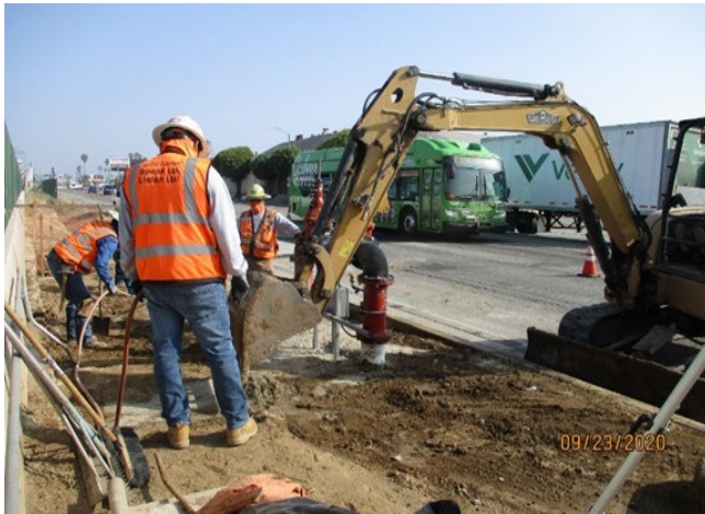
UG1 – Drainage swale grading
