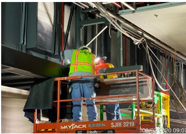
Leimert Park Station- Installing edge lighting at the plaza level.
