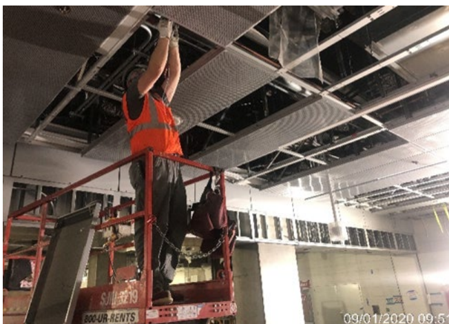
Expo/Crenshaw Station – Modifying and installing ceiling panels.
