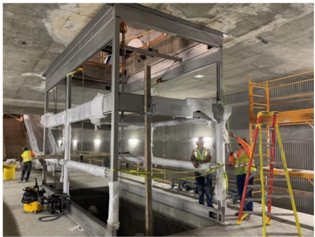
Stainless steel elevator frames at platform level at Historic Broadway Station
