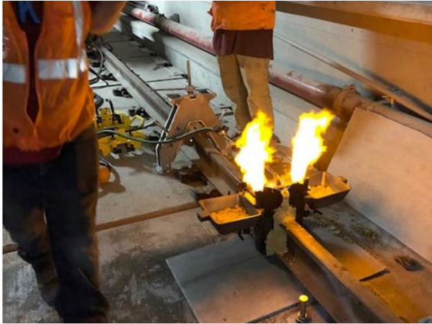
Pre-heating rail for Orgo-Thermite welding
