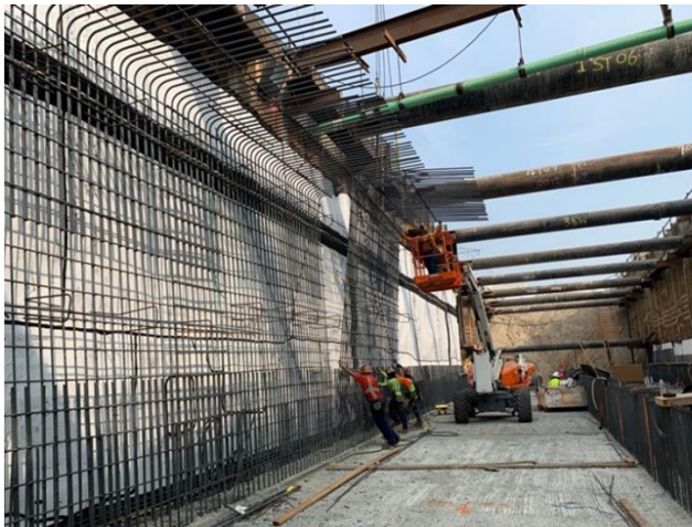
Rebar installation at Alameda Leg
