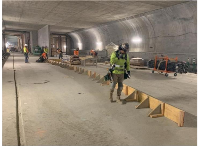
Formwork for DF track in crossover cavern
