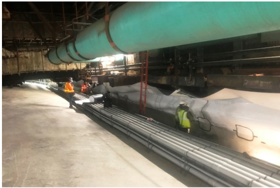
Conduit Installation on Wilshire/La Brea Station Roof
