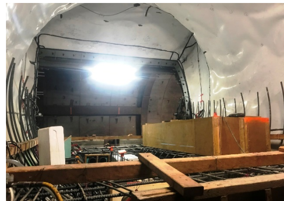
Cross Passage #15 (Reach 1) Formwork Installation
