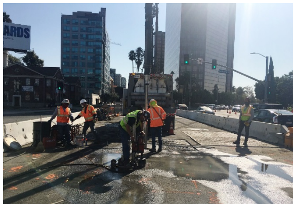
Potholing at Wilshire/San Vicente (Reach 3)
