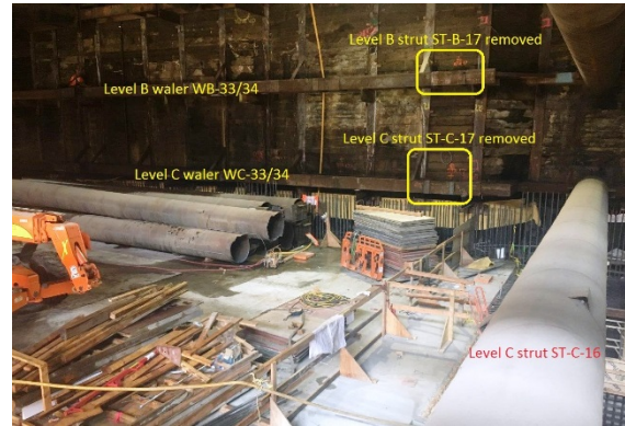
Strut Removal at Wilshire/Fairfax Station
