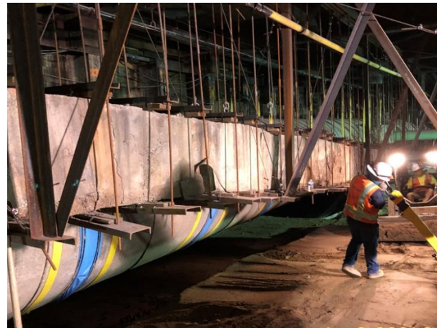
Backfill on Roof Slab 16 at Flower Cut & Cover
