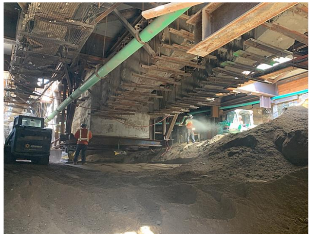
Backfill operations continue at Station Box at Historic Broadway Station
