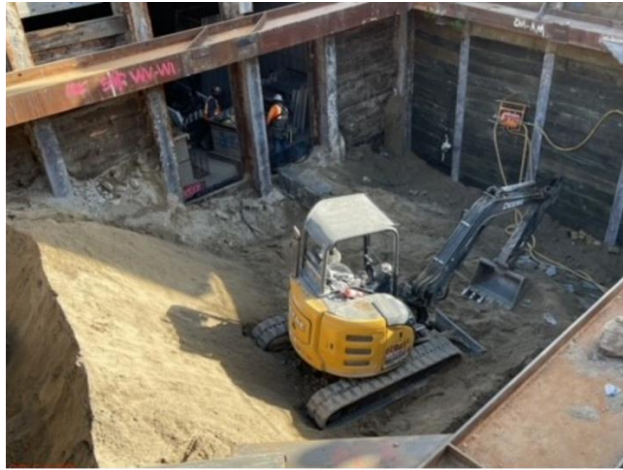
West side structure excavation at future Little Tokyo Station
