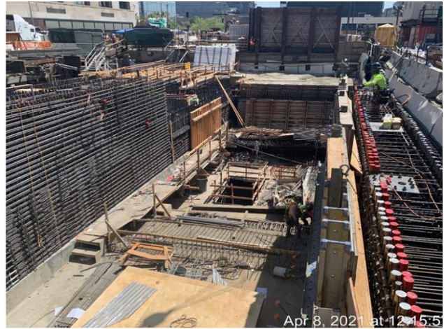
Stem wall formwork at Entrance Structure at Historic Broadway Station
