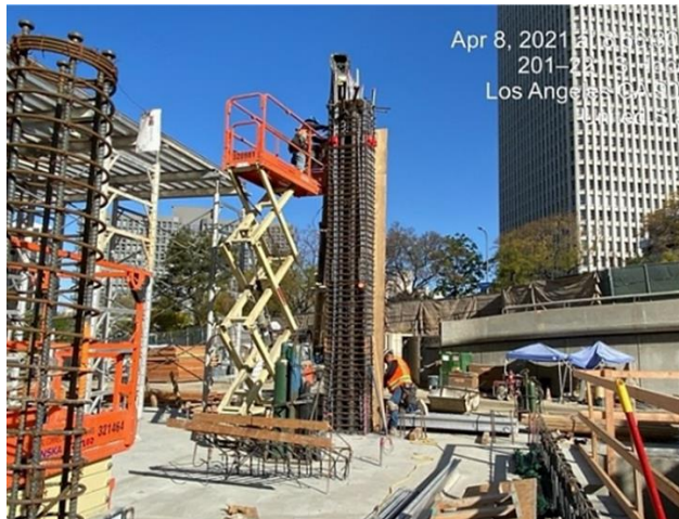
Form installation at Plaza Level of Grand Av Arts/Bunker Hill Station
