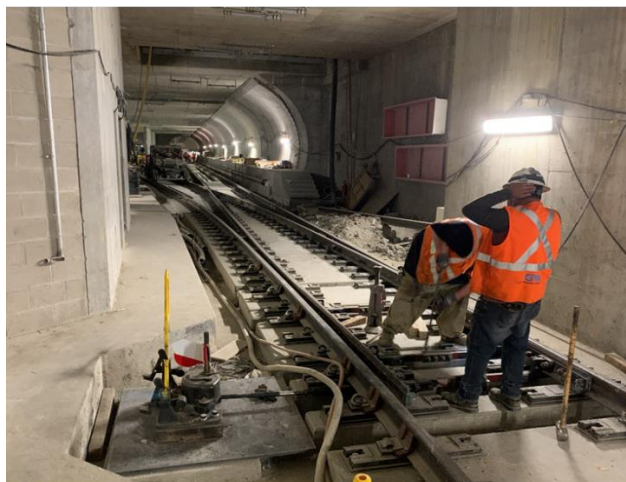
Installing temporary switch at Crossover Cavern
