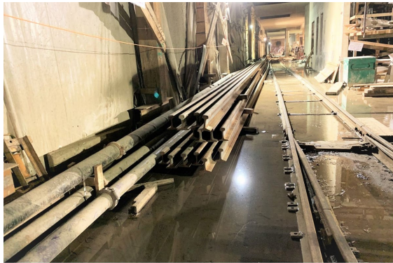
Rail Stored at Wilshire/La Brea Station
