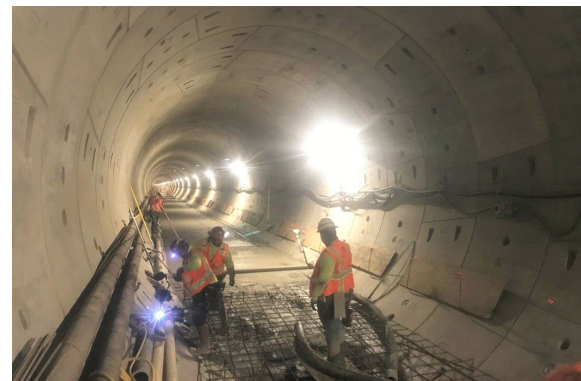
Reach 1 North Tunnel Invert Concrete Placement
