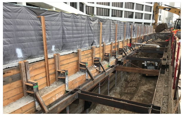
Appendage AE Excavation at Wilshire/La Cienega Station
