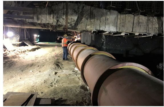
Sanitary Sewer Installation at Wilshire/La Brea Station
