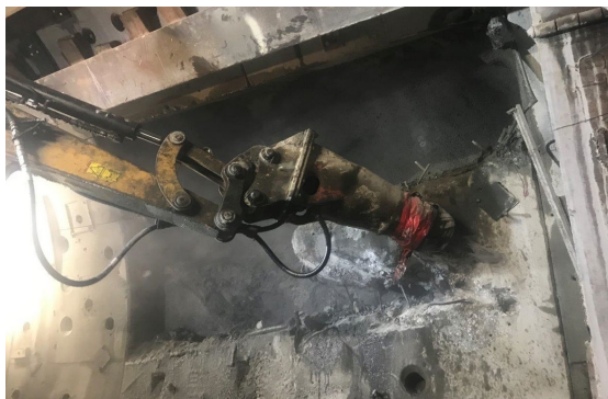
Cross Passage #7 (Reach 1) Excavation
