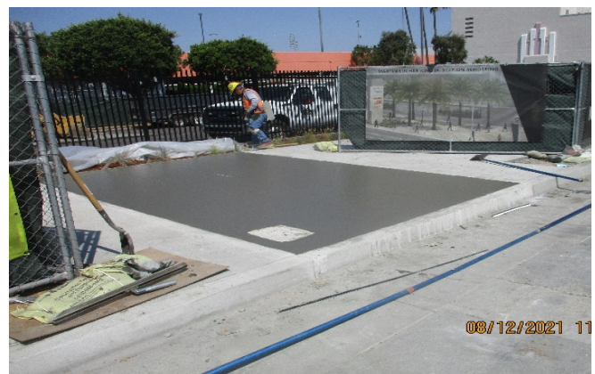
MLK STATION SITE – Placed concrete for sidewalk panel on southbound Crenshaw Blvd between Stocker St and Martine Luther King Blvd.
