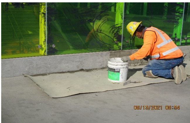
LEIMERT PARK STATION – Sacking and patching the concrete curb around the main entrance plaza canopy.
