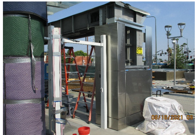
EXPO STATION – Continue stainless steel cladding panel installation to the main entrance roll-up door.
