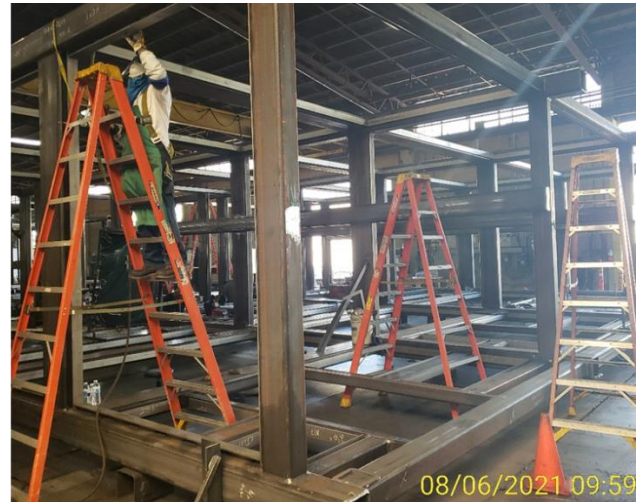
08/06/2021 09:59 Elevator steel manufacturer onsite quality visit
