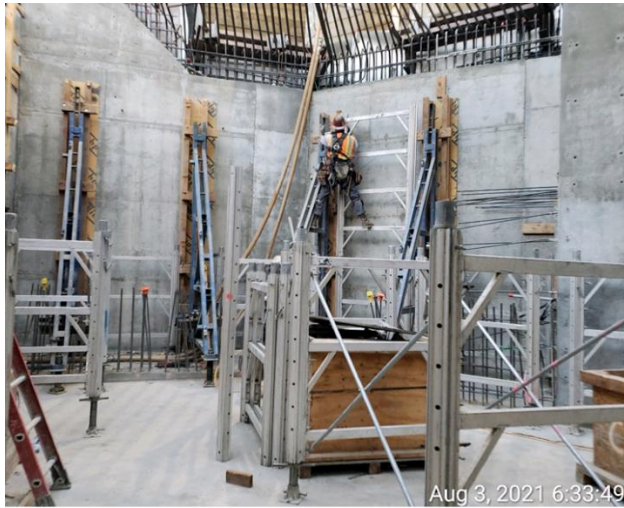
Aug 3, 2021 6:33:49 Shoring towers and roof deck falsework at Fan Plant
