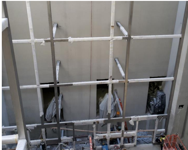
Elevator seat installation at Grand Av Arts/Bunker Hill Station
