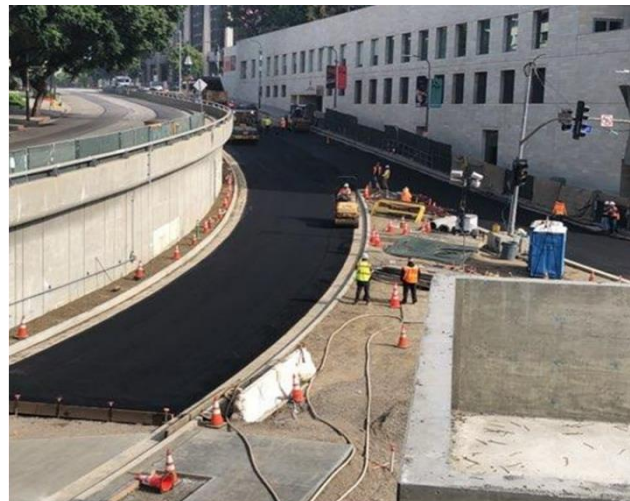
Hope Street pavement operation
