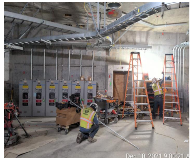
Conduit installation in Wye disconnect room
