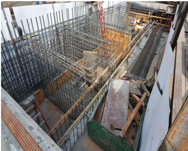
Rebar installation at east vent shaft upper section
