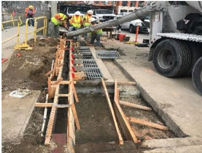
Storm Drain Line A1 Concrete Placement at Wilshire/Gayley
