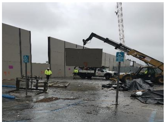
Sound Wall Removal for Upcoming VA Steam Tunnel Relocation
