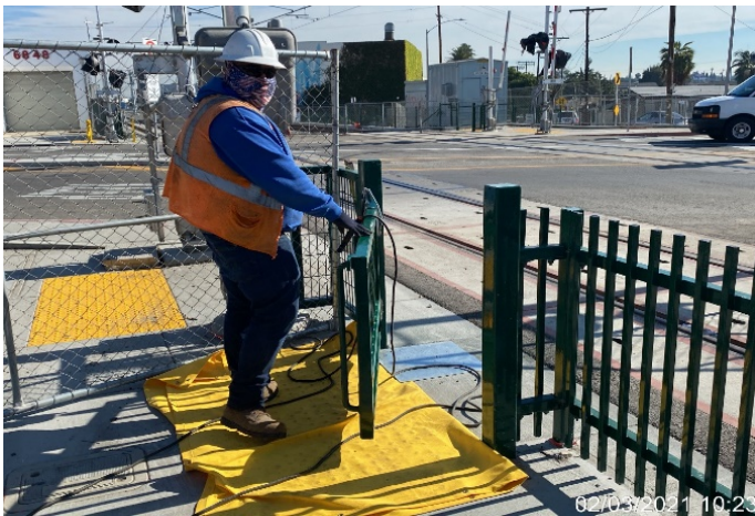
WEST STATION - Ace Fencing installing gate at West station.
