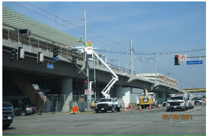
AVIATION/CENTURY - Standing the temporary signal pole at Aviation and Century. Facing NW.
