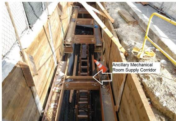
Wilshire/Fairfax Appendage A2A – Wall Form Installation
