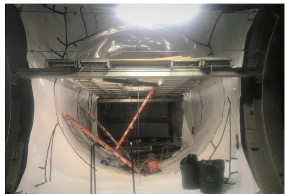
HDPE Installation at Cross Passage #5 (Reach #1)
