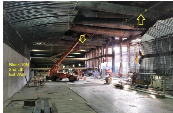
Roof Rebar Installation at Wilshire/Fairfax Station
