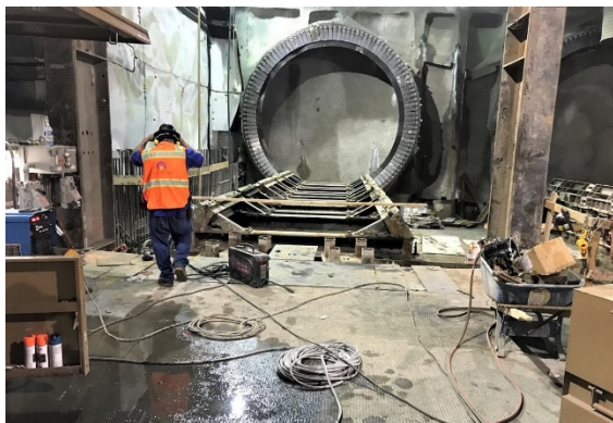
TBM Cradle Assembly at Wilshire/La Cienega Station
