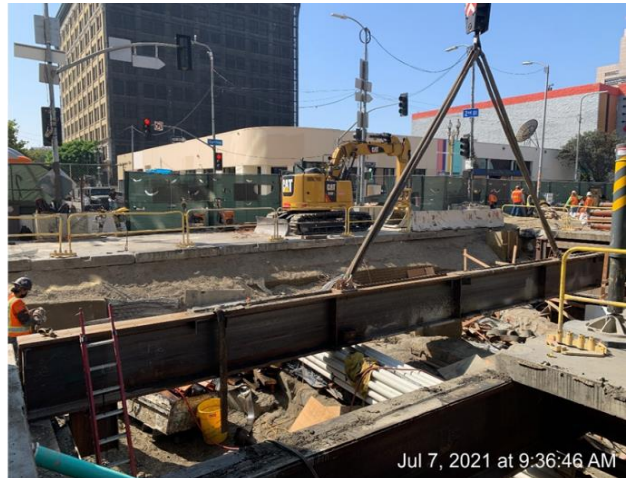
Deck beam 29 removal
