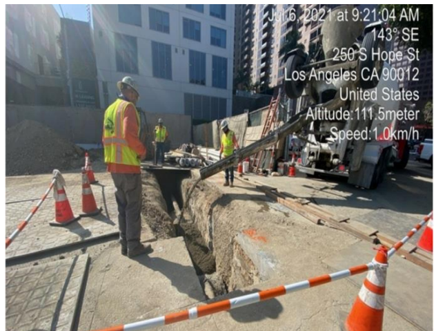
Placing Backfill Slurry Over 6-inch DI DWP Water Supply
