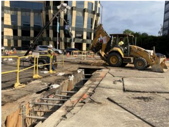
Compaction in Westwood/UCLA Excavated Utility Trench
