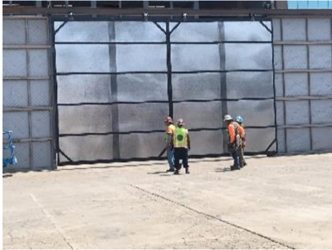
Gate Installed in Sound Wall at Construction Staging Area (UCLA Lot 36)
