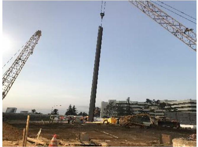
Support of Excavation Piling at I-405 On & Off Ramps
