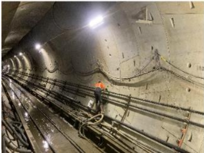
Extending Utilities for Mining Operations for TBM
