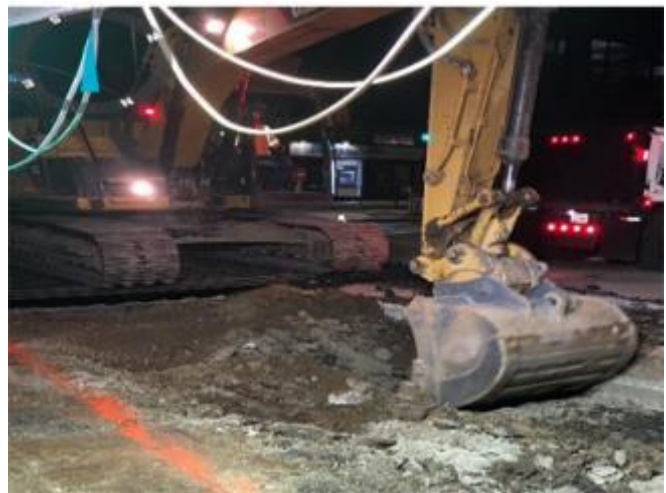
Trench Box Excavation for Storm Drain Line at Wilshire and Gayley
