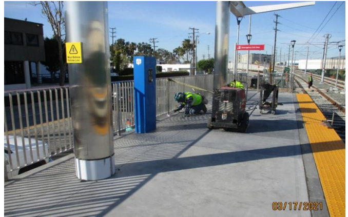
HINDRY STATION – Welding the handrailing at the Hindry Station.
