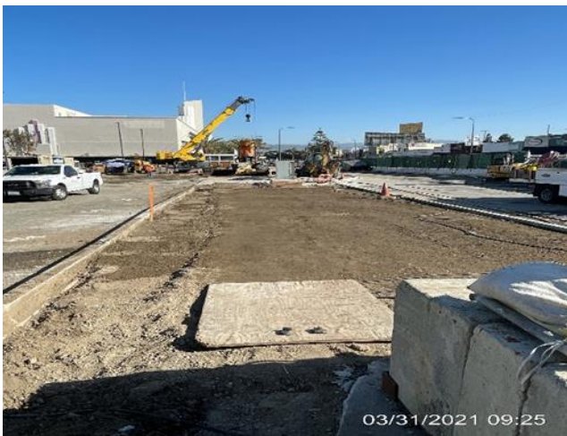
MLK STATION – Backfilling/compacting walkway area on the far south end area.
