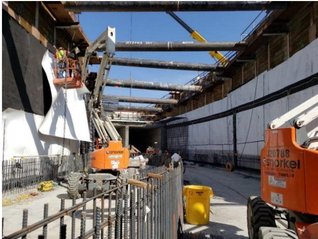
HDPE installation at future Little Tokyo Station
