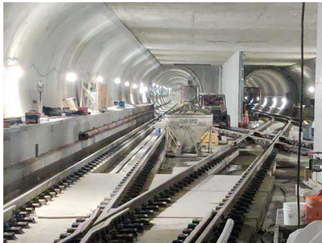
Overview of Crossover Cavern adjacent to Historic Broadway Station
