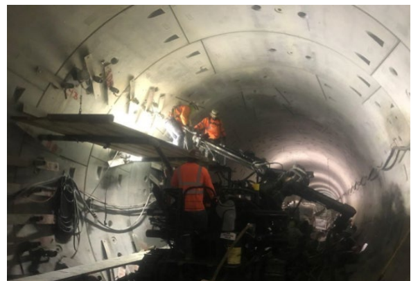
Grouting Operation at Reach 2 Cross Passage #16
