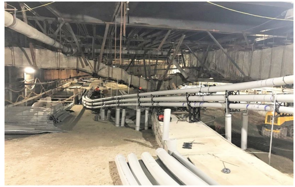
Wilshire/La Brea Station Duct Bank Installation Above Roof
