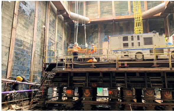
Transporting Material from Wilshire/Western Shaft
