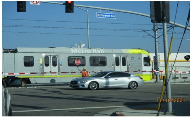
HINDRY STATION – Flagging for train testing at the Hindry crossing. Facing north.
