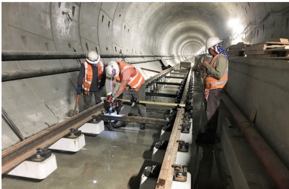
Trackwork Installation in the Reach 1 North Tunnel
