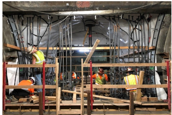
Rebar Installation at Cross Passage 20 (Reach 2)
