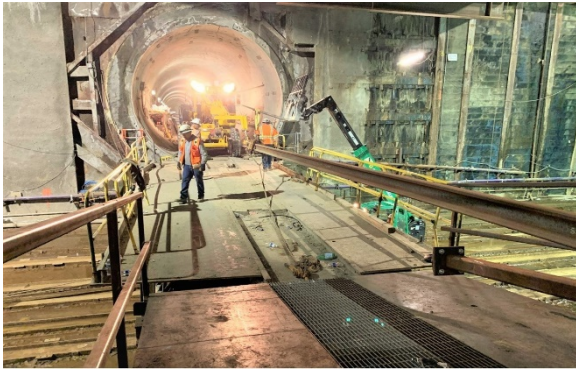
Delivery of Rail from the Division 20 Yard
