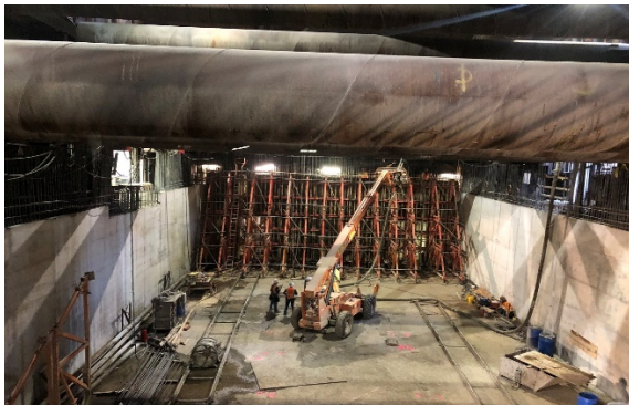
West Hammerhead Exterior Wall at Wilshire/Fairfax Station
