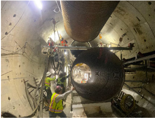
Testing and Commissioning of TBM "Aura" in the BL Tunnel
