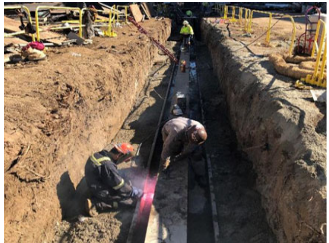
UCLA SOE Welding Cap Beam to Cap Water
