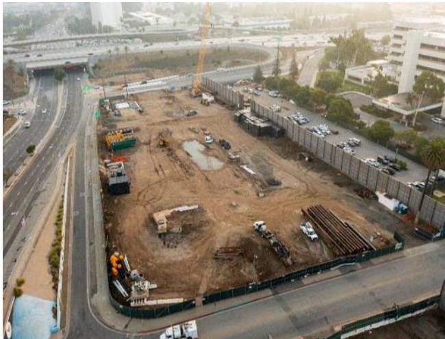
Westwood/VA Station Overview
