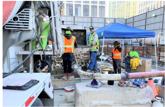
Pumping Concrete to Support Reach 1 Tunnel Operations
