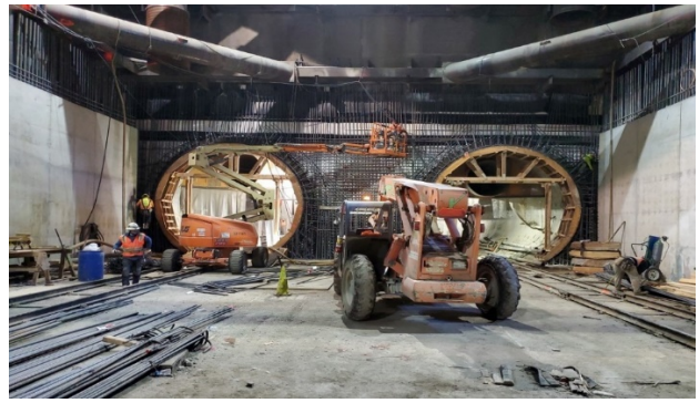
Hammerhead Rebar Placement at Wilshire/Fairfax Station
