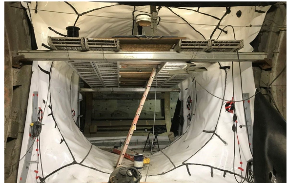
Waterproofing at Cross Passage 20 (Reach 2)
