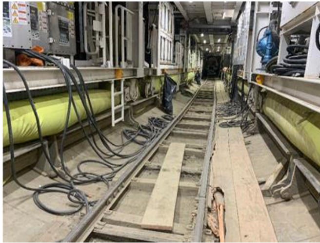
Cable and Wiring Installation for BL "Aura" TBM
