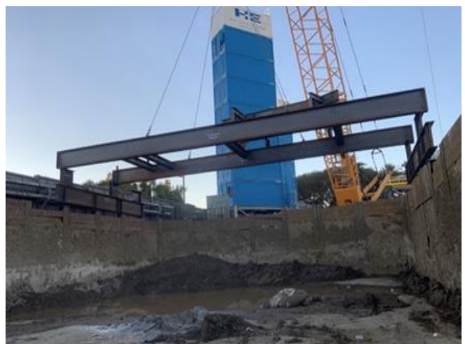
Muck Pit Dump Assembly
