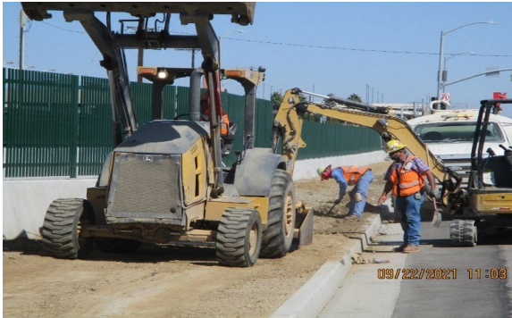
AVIATION STATION – WSCC grading sidewalk at Aviation
