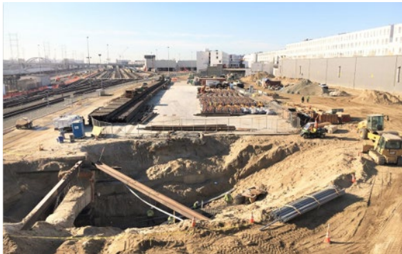
Track & Block Delivery at the Division 20 Yard
