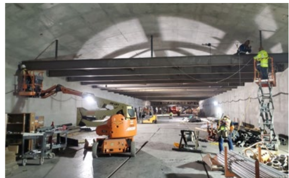
Plenum Steel Installation at Wilshire/Fairfax Station
