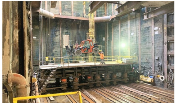
Hoisting Equipment through the Wilshire/Western Shaft
