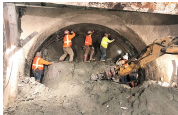
Excavation at Cross Passage #16 (Reach 2)
