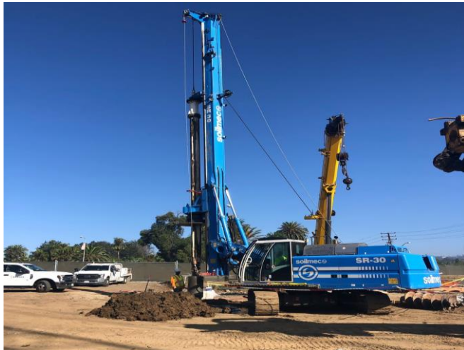
Drilling Dewatering Well at VA Lot 36
