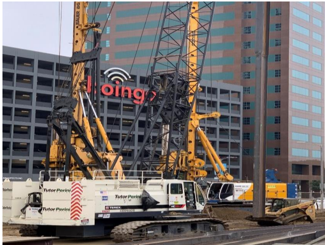
SOE Pile Installation for Westwood/UCLA Station
