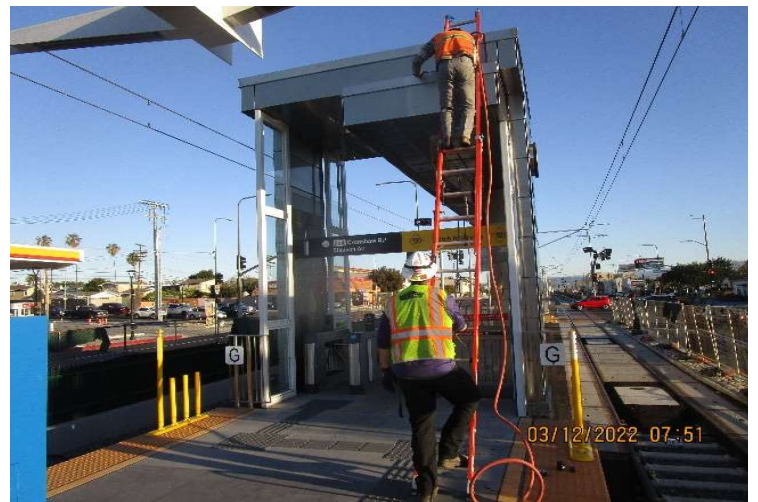
HYDE PARK STATION – Performing water pressure testing for the roof drains at the south pavilion.
