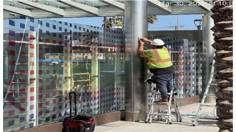
EXPO STATION – Applying anti-graffiti shield to the main entrance canopy columns at the plaza.
