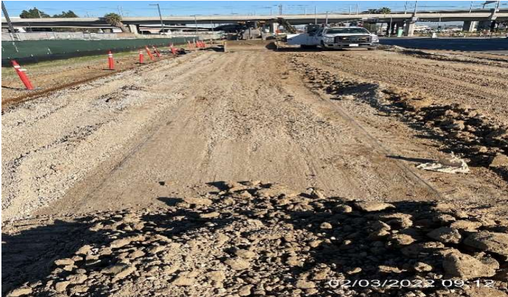
AVIATION STATION – WSCC removing steel plates from job site at Aviation/118th
