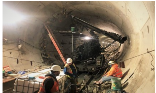
Ground Mitigation at Cross Passage 25 (Reach 3)
