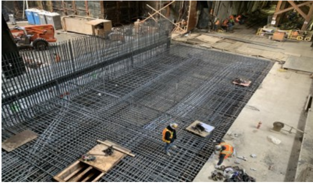
Invert Rebar Installation at Wilshire/La Brea Station
