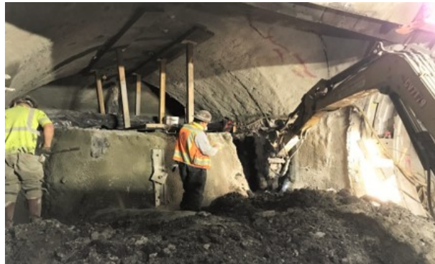
HDPE Installation at Cross Passage 21(Reach 2)
